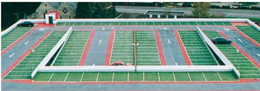
BASF Construction Chemicals' solutions for car park top decks provide exceptional tensile strength and elastomeric capability. Double the thickness of most products, they use a multi-layer build up system to ensure optimum performance in even the harshest environments. Spray application speeds up the installation process and gives controlled thickness.
