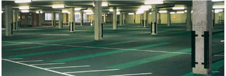
Light-reflective coatings can be applied to the walls, soffits and columns of lower decks to improve aesthetics by exploiting ambient light and headlight beams. The result: brighter and more secure car parks, and a reduced need for additional lighting installations.
