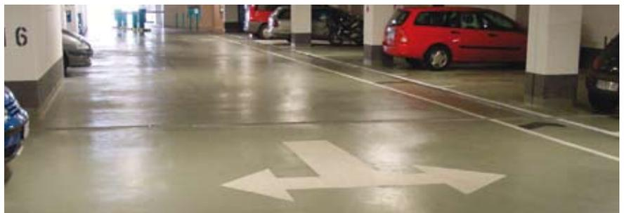
For decks, top coats are available in a choice of colours, helping users to identify different areas of the car park with ease. Skid resistant finishes are available to give extra grip, reduce tyre squeal and to provide a sure footing for pedestrians.
