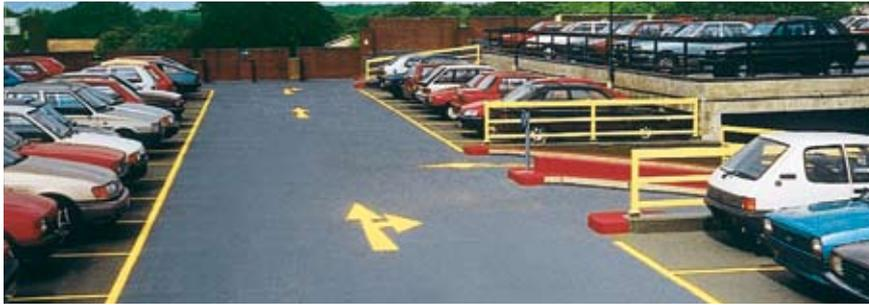
One specification of product across an entire parking structure is unlikely to be the best solution for all areas. The top deck of a car park is the structure's most vulnerable surface, exposed to the elements as well as to oils, acids, salts and UV radiation. To withstand such severe conditions, heavy-duty, UV-stable, elastomeric waterproofing systems are needed.
